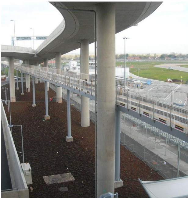
Compare lightweight PRT guideway (top-left to bottom-right) with large elevated roadway (top)
