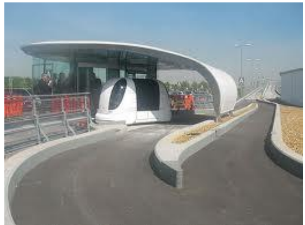
Vehicles can easily bypass any stations where a stop is not required. These 'offline stations' allow nonstop service from origin to destination, without intermediate stops.
